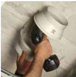
Fix the support bracket.
