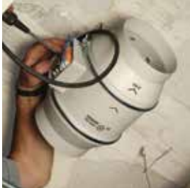
Carry out the wiring connections.
