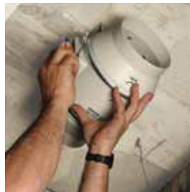
Place the impeller and motor assembly.
