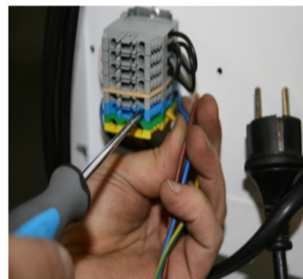
5 Connect power and remote humidostat wires.
