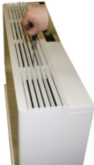
1 Unscrew casing's screw.
