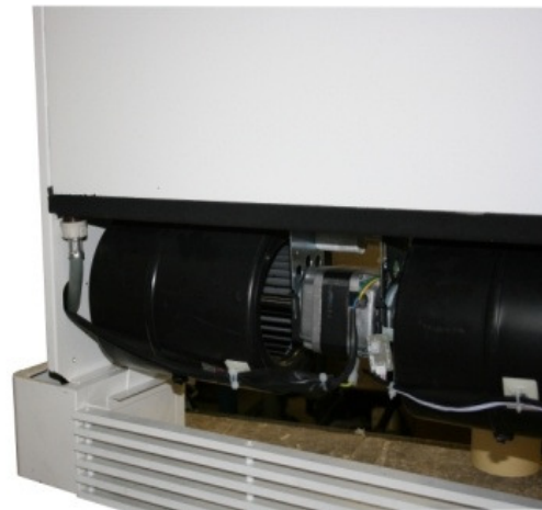
5 Connect power and remote humidostat wires.
